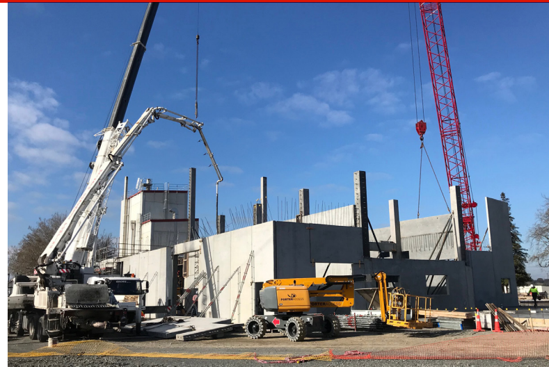
Construction of the $50 million industrial sprayer should be completed by February 2020.
